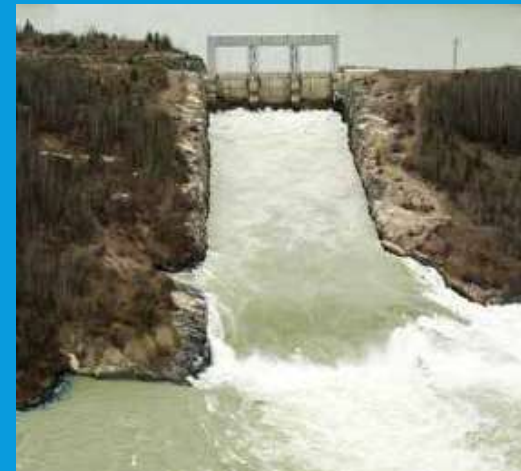
Notigi Control Structure Source: RCEA Summary Report, p. 19
