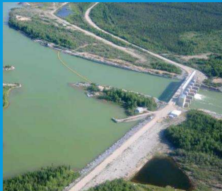
Missi Falls Control Structure Source: RCEA Summary Report, p. 31
